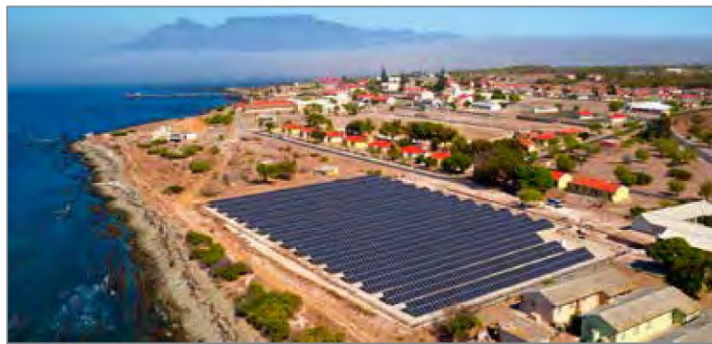
Photograph provided by ABB
